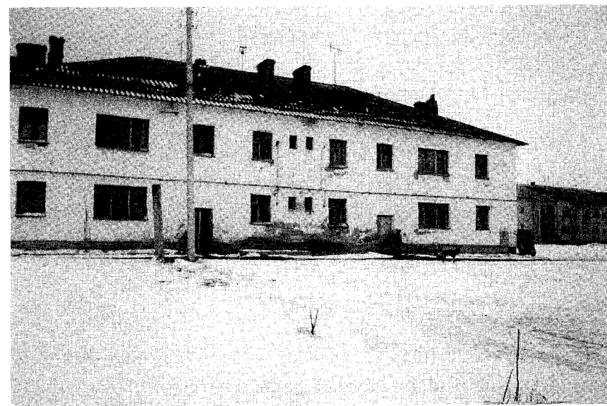
29. At Verchnyua Troitsa, one of the new village's two-story houses, each containing sixteen flats
